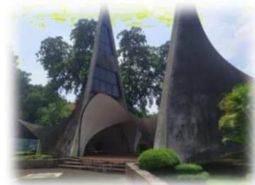
Gambar 1.5 Atap DaK Beton
