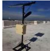
Gambar 3. 14 PJUTS solar Tracking
