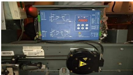
Gambar 3.9 Inverter BG202-XM.
