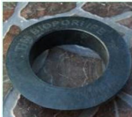
Gambar 6. Ring baja penguat mulut biopori
